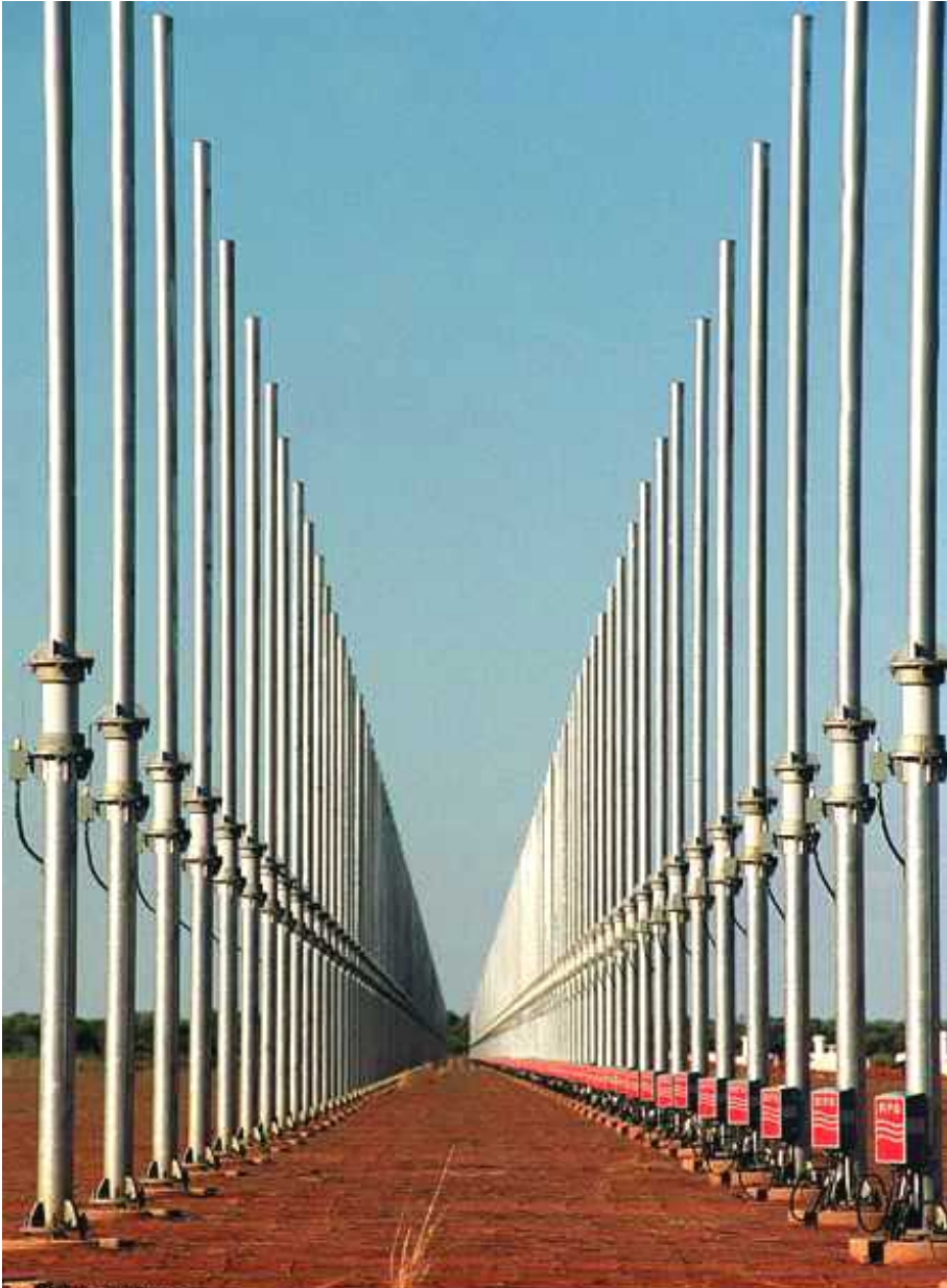
FIGURE 1.10. Over-the-horizon radars operate by refracting HF radio waves from the ionosphere; they typically use antenna array kilometres in length. The figure shows one of the Australian Jindalee radar receivers.
